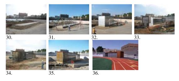
An array of steel components (weathering Cor-Ten, structural tubes and connectors, galvanized corrugated decking, porcelain and perforated screens) were assembled to produce varying patterns of transparency and opacity and to differentiate the porcelain steel half-time huddle "chalk board" privately facing the home-team school building, the operable storage door-wall facing the field, and the concession stand east of the portal (*figures 37-39*).
